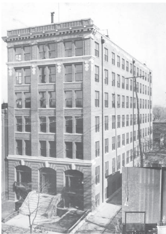
The Bureau of Chemistry laboratory building (left) and the drug inspection laboratory inside (below).
